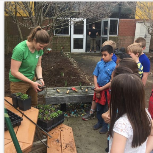
Courtyard garden installation to prevent runoff
