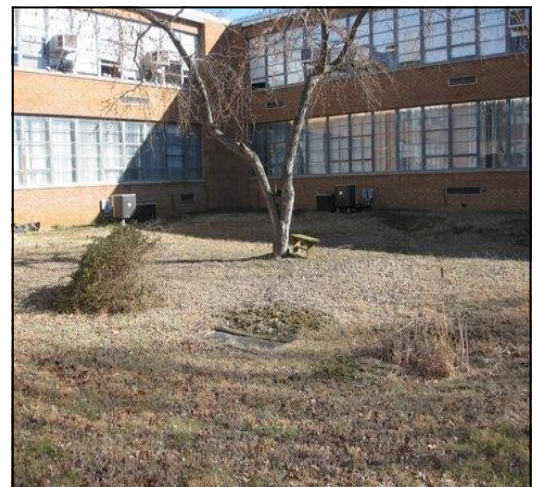
"Before" courtyard condition, all mowed grass to drainage system.
