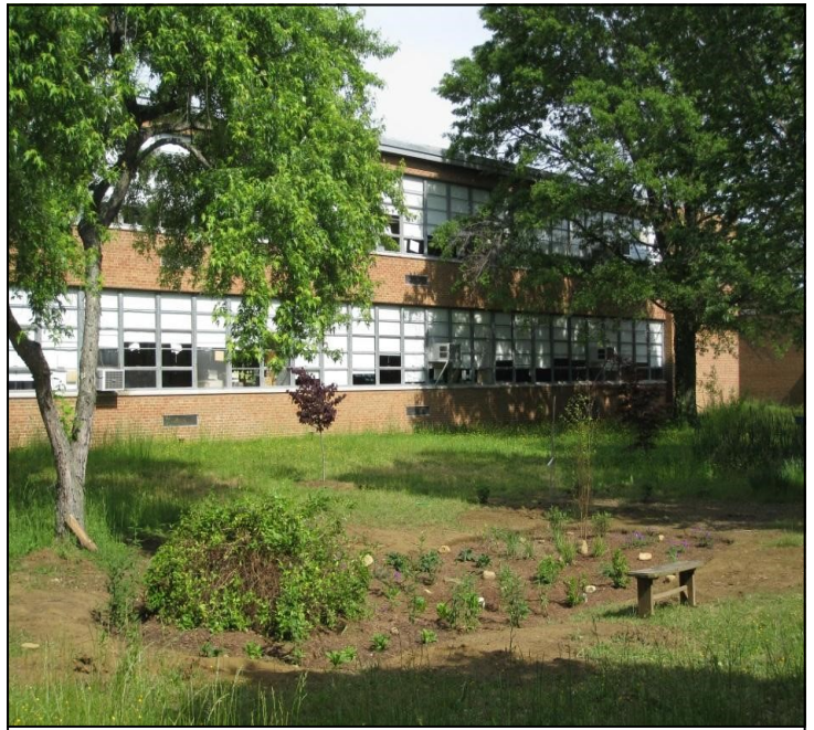
Newly planted rain garden and native understory trees, which have continued to thrive.
