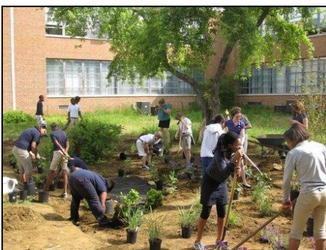
7 th graders installing the rain garden
